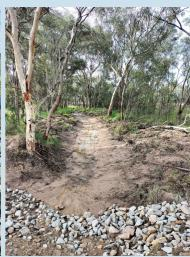
Part of this work involved repairing the work that we had done a few years ago along Henley road, the photo shows how the drain had deteriorated with vehicles driving over it.
